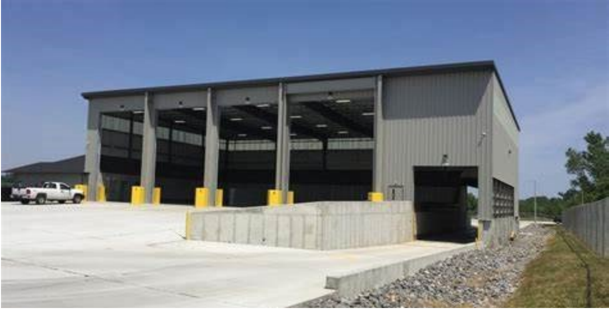
Figure 3 - Transfer station City of Greensboro, NC
