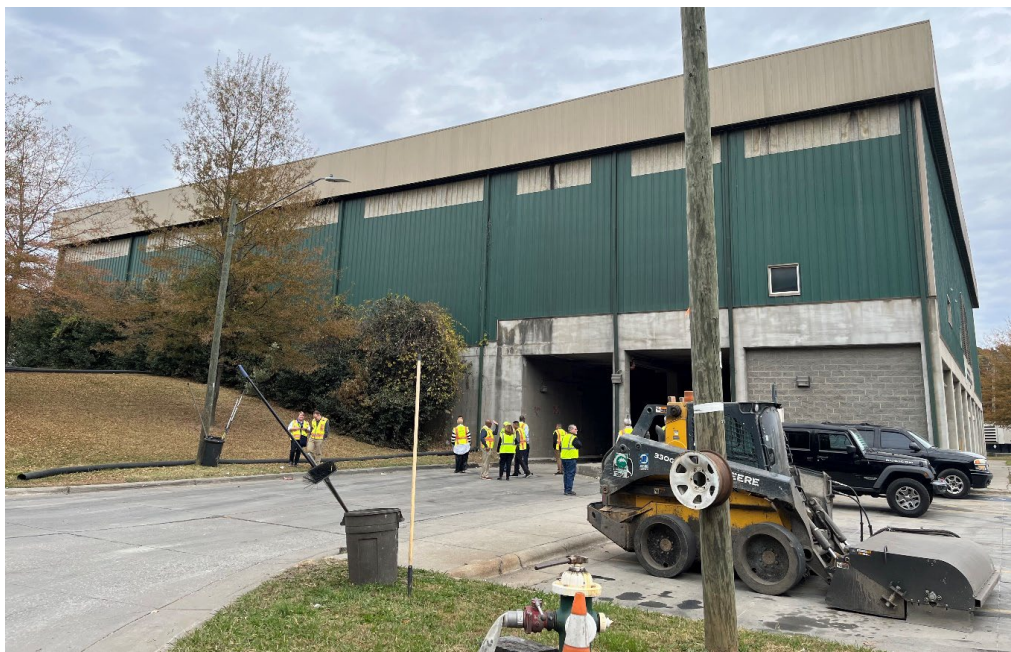
Figure 2 - Transfer station City of Greensboro, NC
