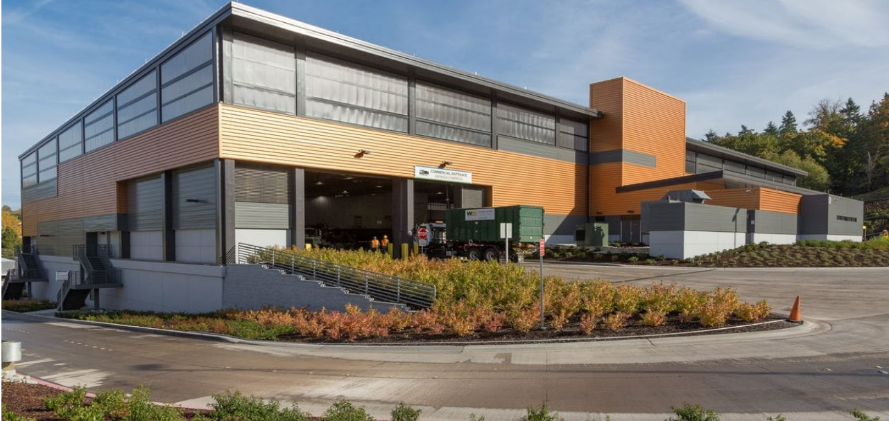
Figure 6 - Factoria Transfer Station, King County, WA
