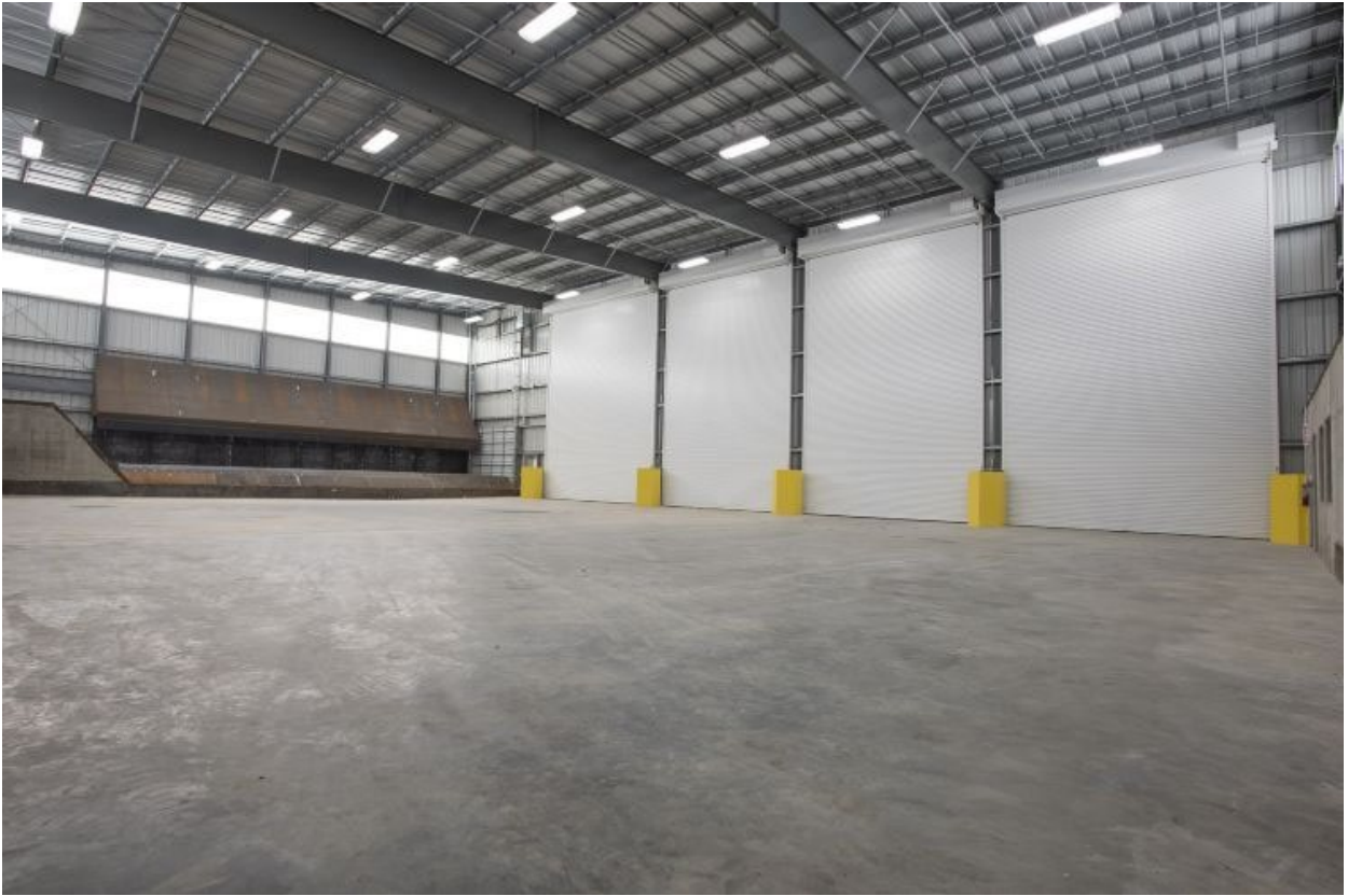
Figure 4 – Interior view transfer station Cape Girardeau, MT
