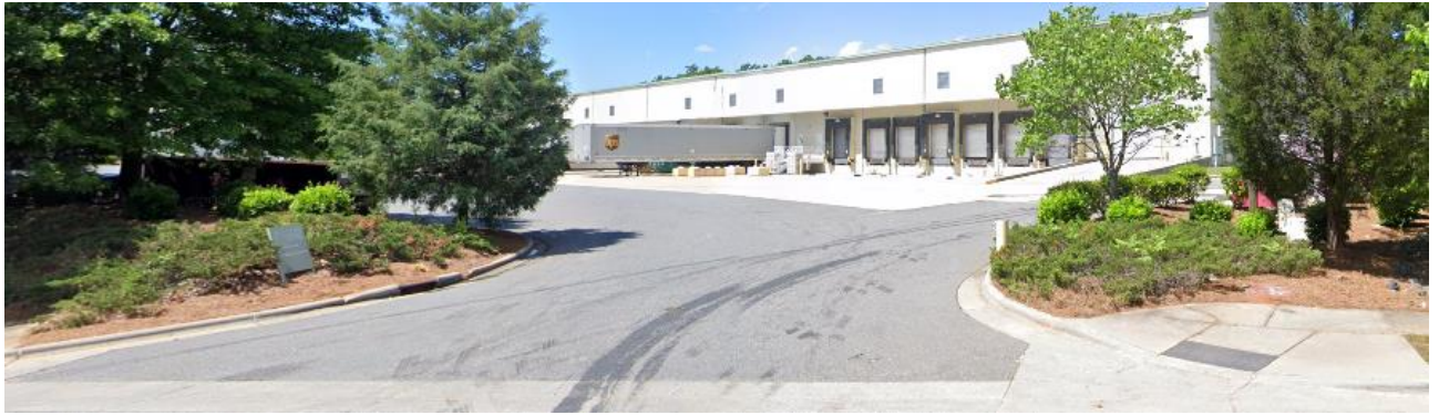
The property to the north is developed with warehouse/distribution uses.
