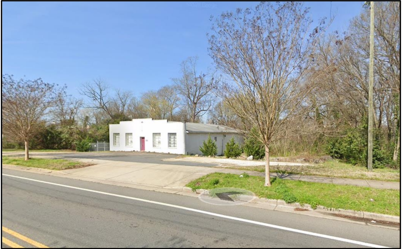
Streetview from Seigle Avenue looking east toward the subject property. The structure in the background of the photo will be adaptively reused as a part of this project.
