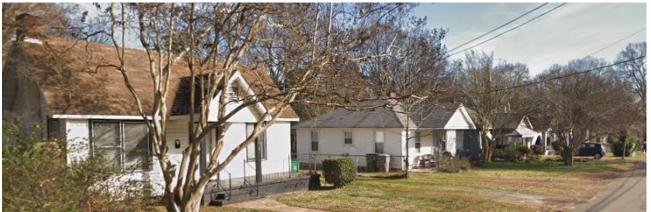
The properties to the west are developed with residential uses.
