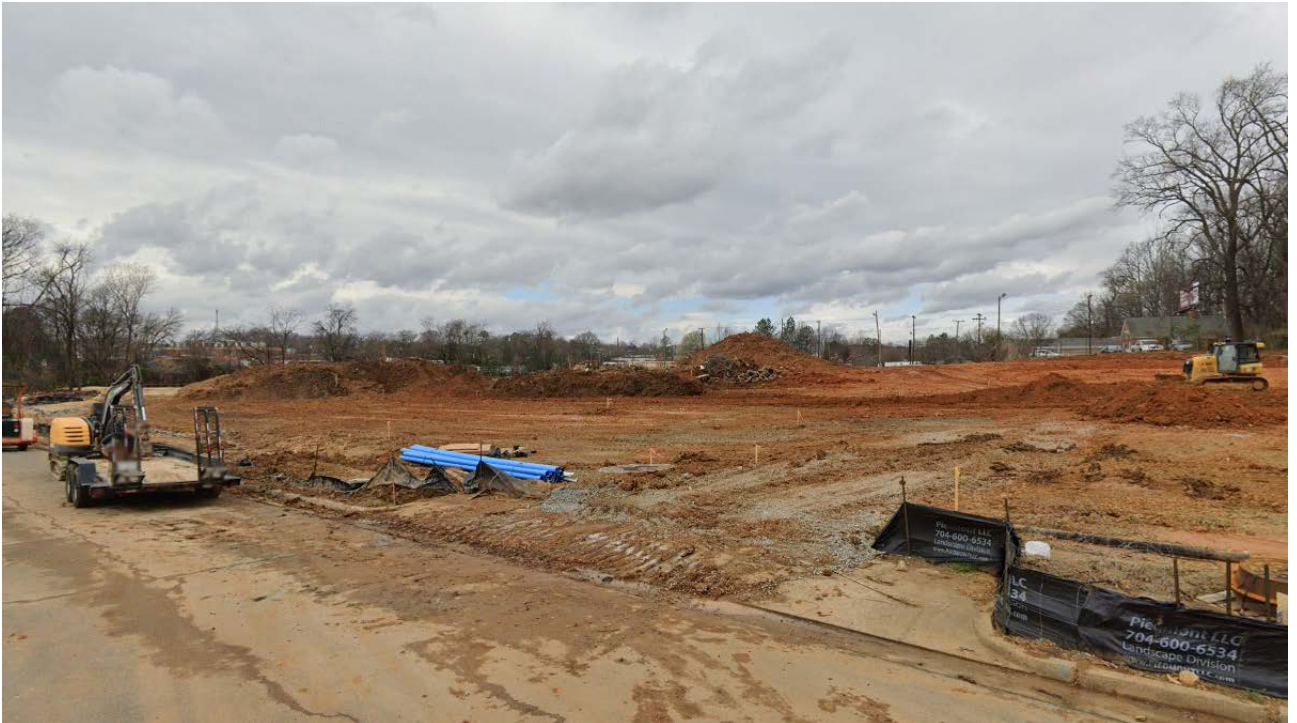
View of the property's frontage along Benard Avenue, a dead end street that historically served light industrial-type uses. Amelie's new location is located just outside the frame to the right.
