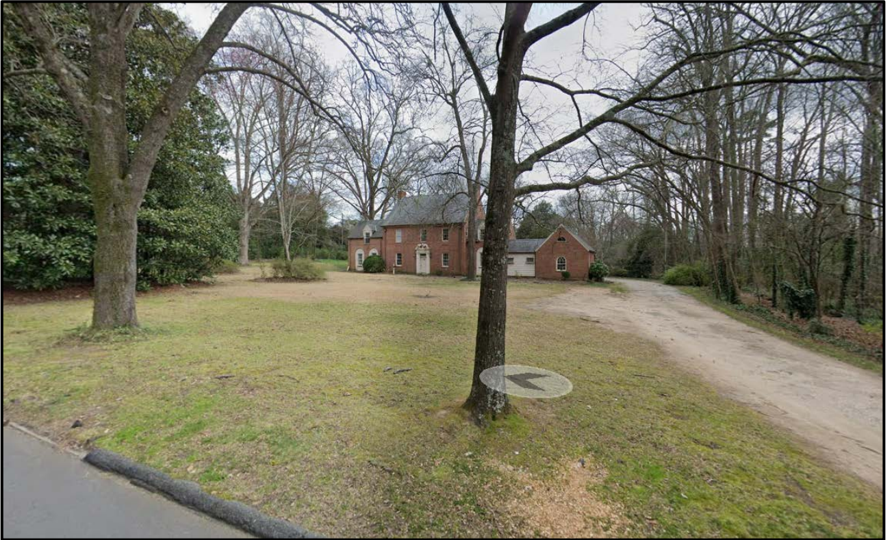
Streetview from Mecklenburg Avenue looking southeast toward the subject property. The Shaw House can be seen in the background and would be rehabbed with this petition.
