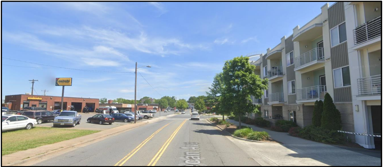
The site is adjacent to commercial and residential uses to the north along Pecan Avenue.
