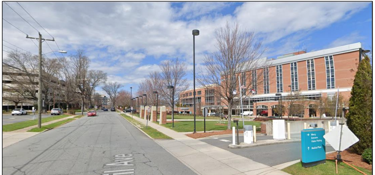
The rezoning site is immediately surrounded by medical office buildings and health institutions.
