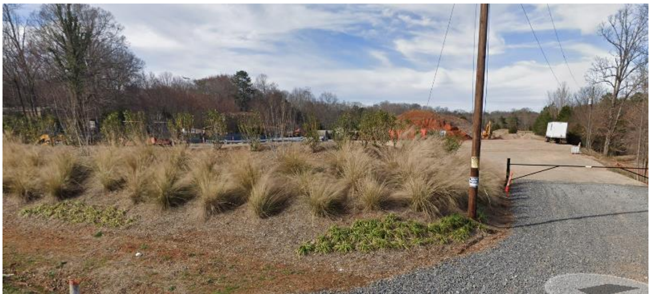
The property to the west is under construction for industrial uses.
