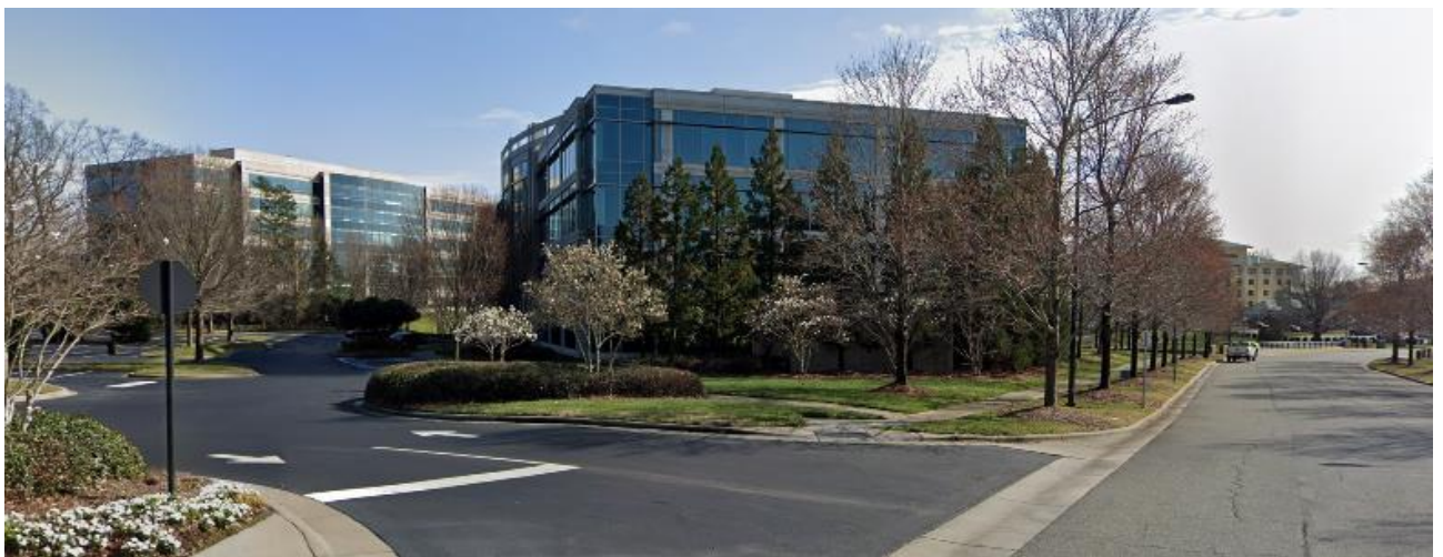
The properties to the south are developed with office uses.
