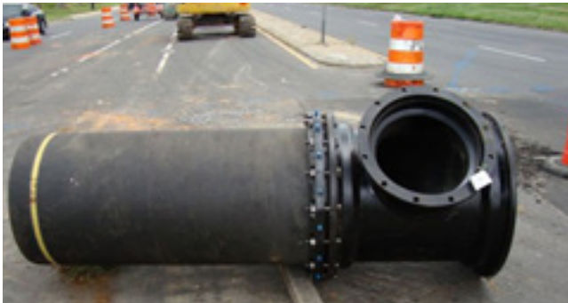
Cast Iron (CIP) & Ductile Iron (DIP) – frequently used for large transmission and distribution mains. Ductile iron pipe is 95% recycled material.
