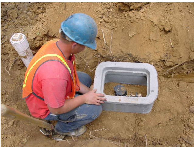
Meter and meter box installed for a new customer.
