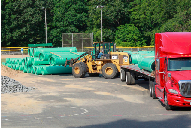
24-inch wastewater pipe being delivered to a staging area.
