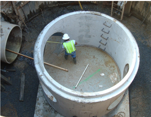
Manholes vary in size depending on the amount of wastewater a community creates.
