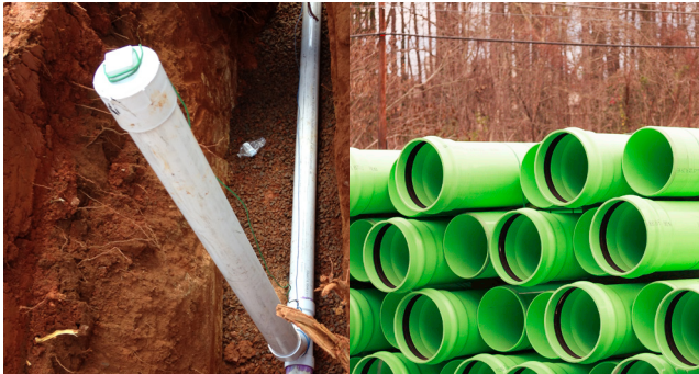
Polyvinyl Chloride (PVC) – largely used for small pipe projects. Roughly 50% of the drinking water system is pvc pipe. Wastewater pipe may be blue or green.
