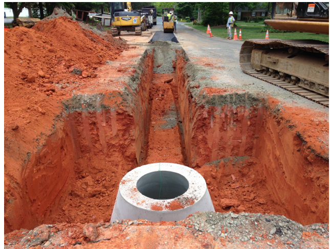
Manholes vary in size depending on the amount of wastewater a community creates.
