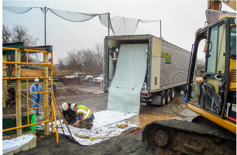
Large diameter pipe rehabilitation project.
