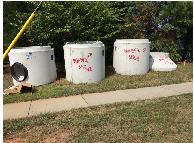
Manholes in road right-of-way beside construction area.
