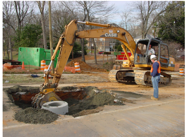
Manhole and wastewater pipe installation for apartment complex.
