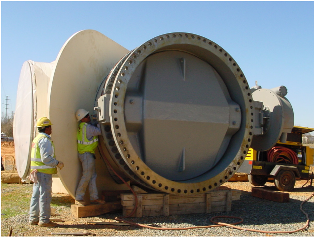
96-inch transmission water main valve.
