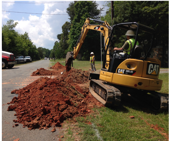
Soil in the road right-of-way.
