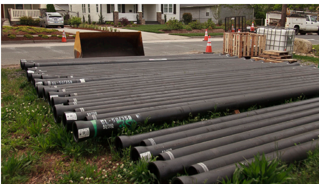
48-inch drinking water pipe delivered to a construction area.
