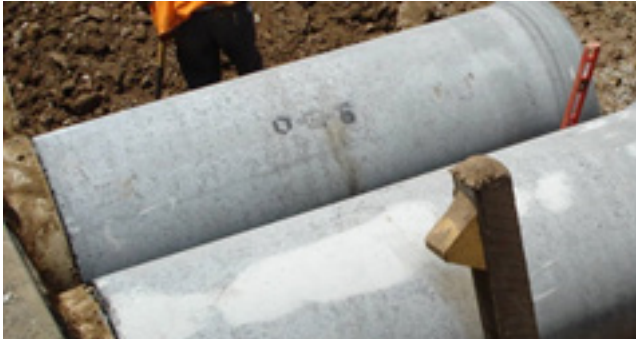
Concrete (Prestressed Concrete Cylinder Pipe, Concrete Cylinder Pipe, and Reinforced Concrete Pipe) – durable older pipe.
