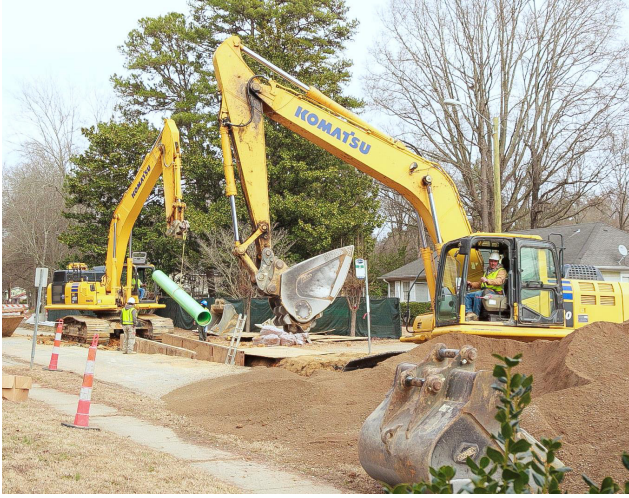
24-inch wastewater pipe project under a street.
