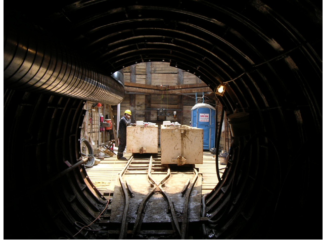
View from inside the tunnel looking at the entry pit.
