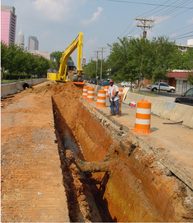
24-inch drinking water pipe installation.
