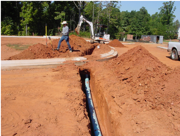
Drinking water installation for a new neighborhood.
