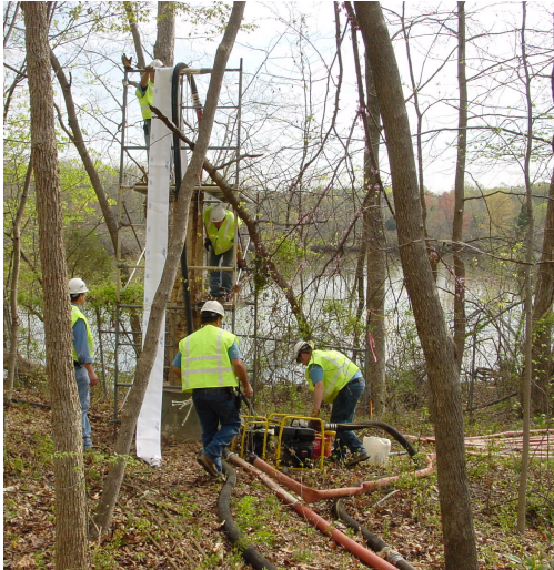
Regular diameter pipe rehabilitation project.
