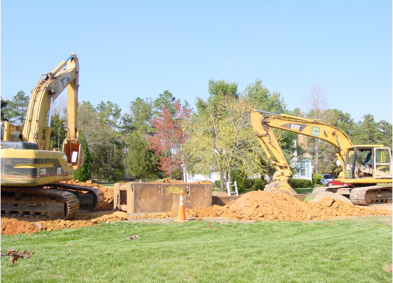
Water pipe extended along street to serve new customers.
