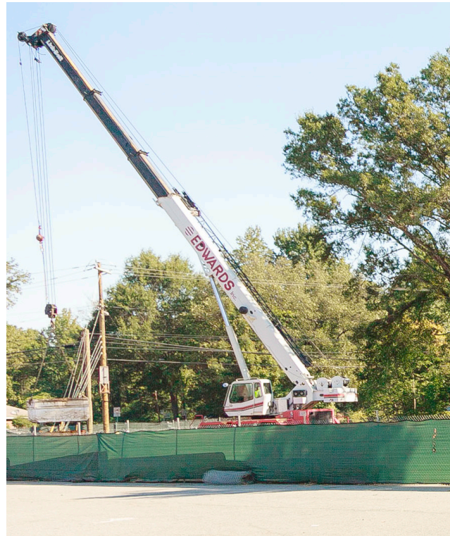
Cranes may be required to move equipment and dirt.
