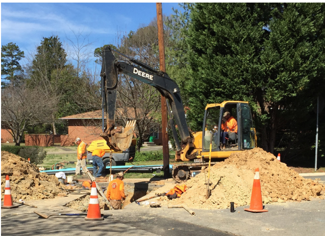
Crews installing new pipe to replace older pipe.
