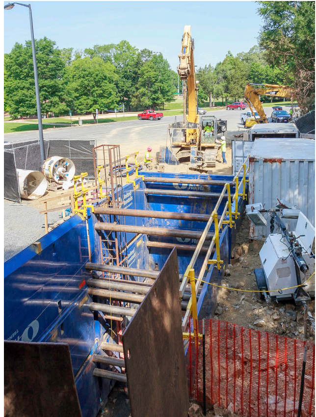
Entry pit to tunnel under a road.
