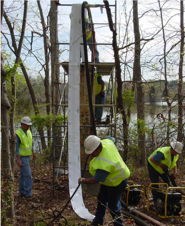
Crew installing new lining in wastewater pipe.
