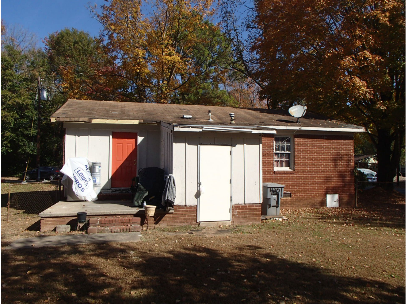
Photo 3 – House – Side C
