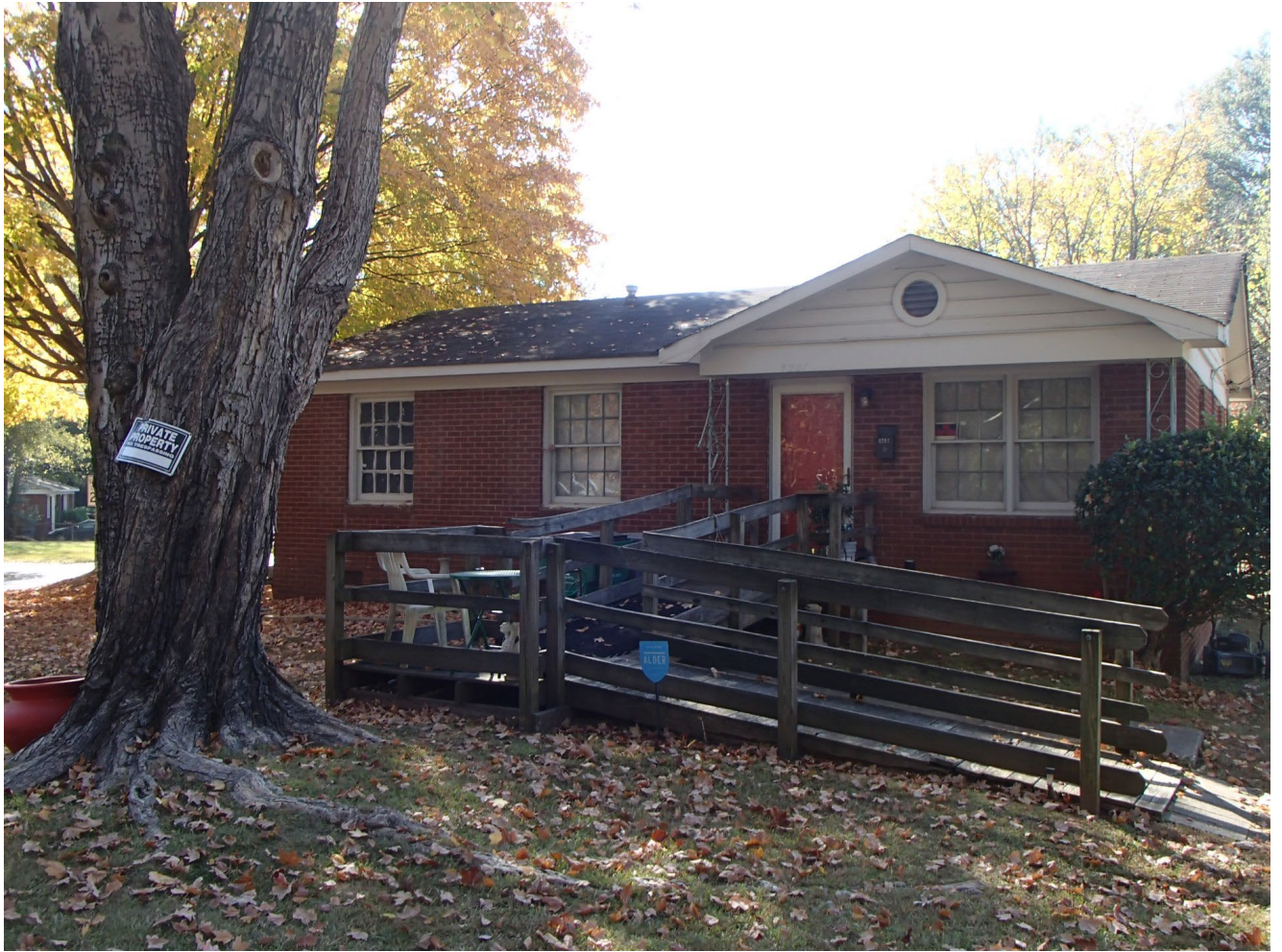
Photo 1 – House – Side A
