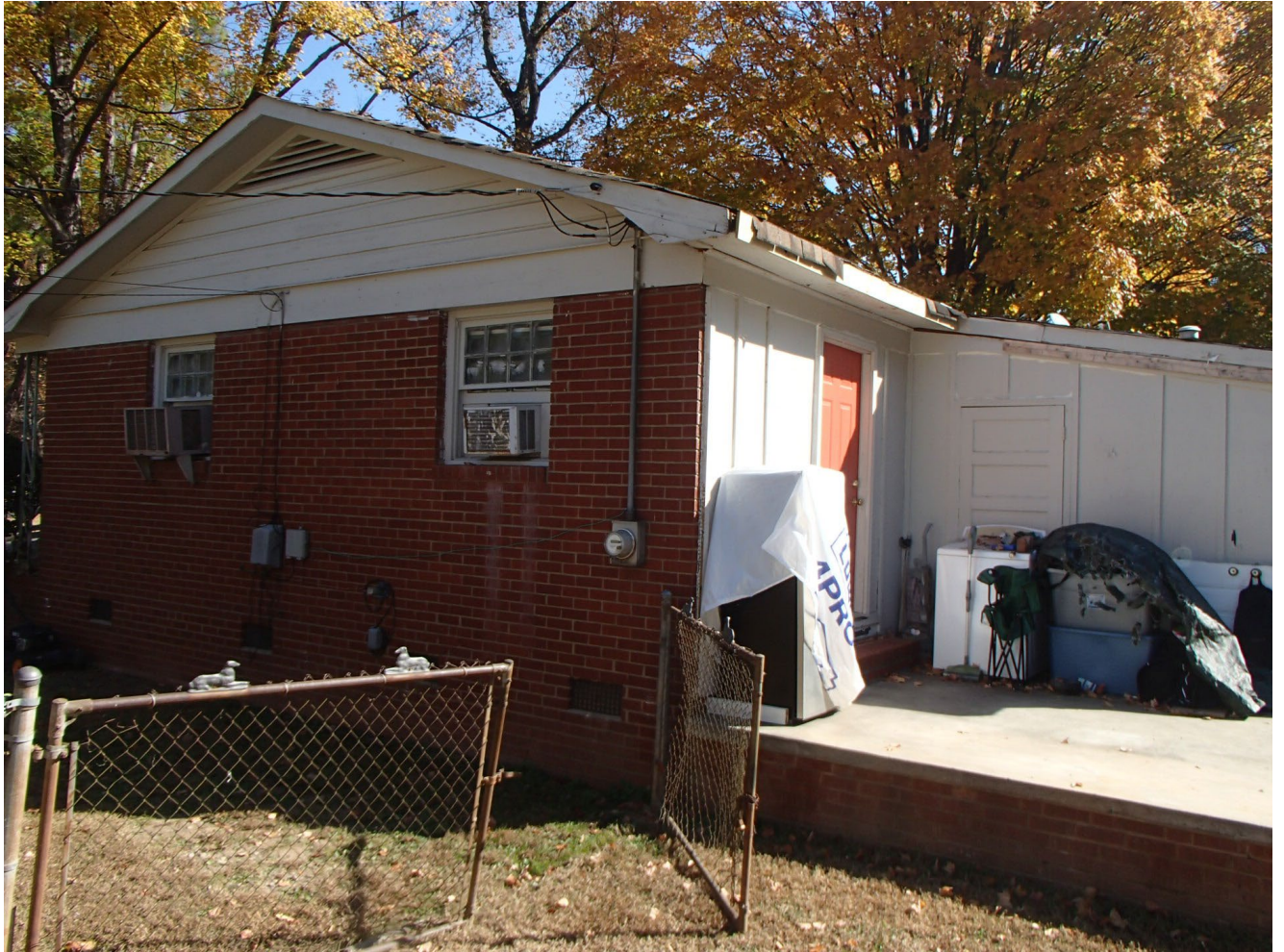
Photo 4 – House – Side D
