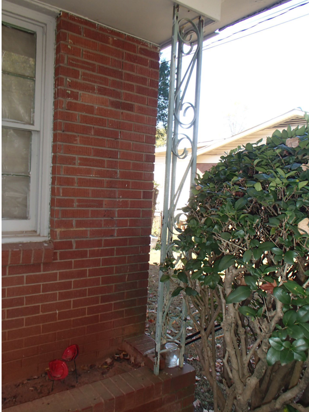
Photo 5 – Side A Ceiling/Overhang and Support Column
