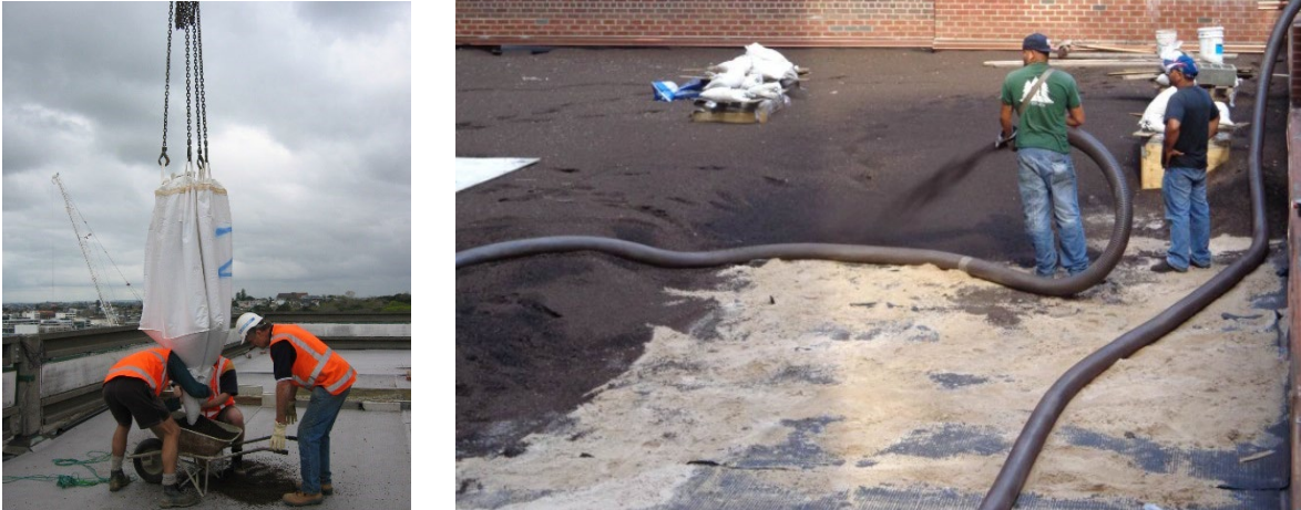
Figure 11. Growing media installation by crane hoist (left) and pneumatic blower (right) (Dr. Elizabeth Fassman)
