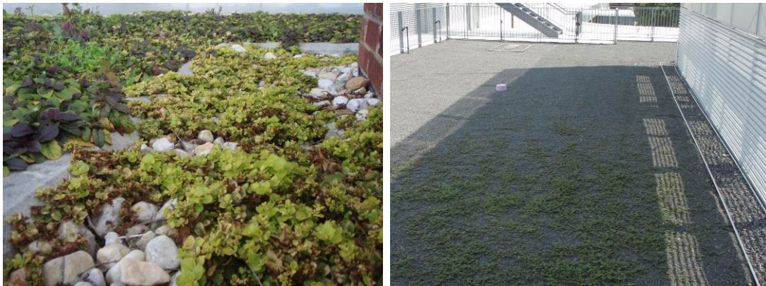
Figure 12: Common Weeds on North Carolina Green Roofs (left) Creeping Jenny likes the hot microclimate of gravel edging. (right) Spotted spurge invades the growing media whose planting has been delayed. (Dr. Elizabeth Fassman)
