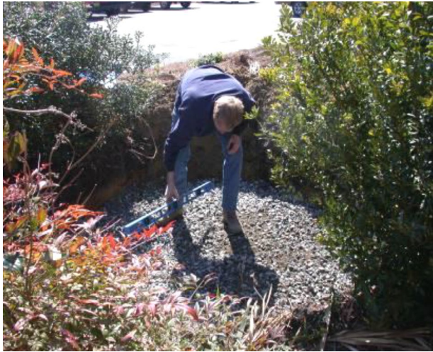
Figure 10. Preparing a cistern footing of aggregate (left) and a concrete footing for a cistern exceeding 1,500 gallons (right) (NCSU BAE)
