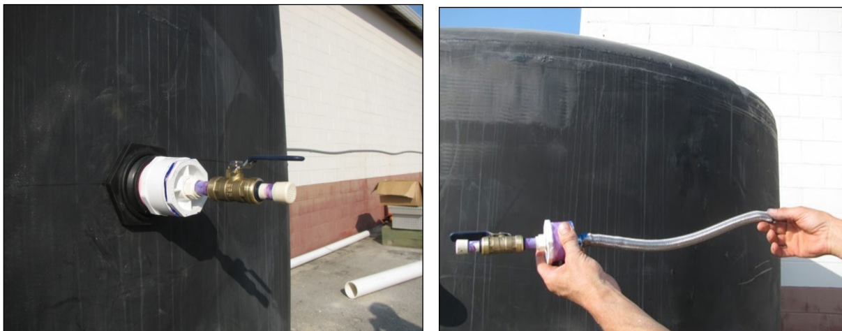
Figure 5. Anti-Clogging Passive Drawdown Mechanism (NCSU BAE)
