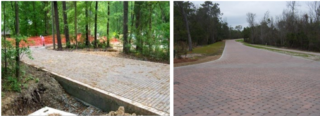
Figure 5. Edge Restraints on PICP
