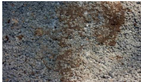
Figure 15. Clogged Pavement
