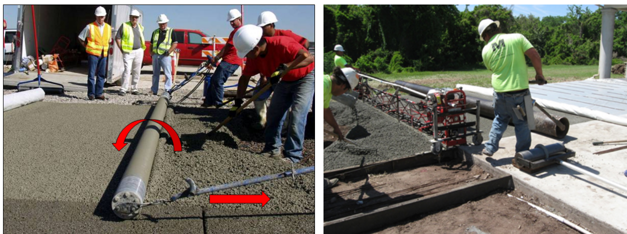
Figure 14. Compacting Pervious Concrete (NCSU-BAE)
