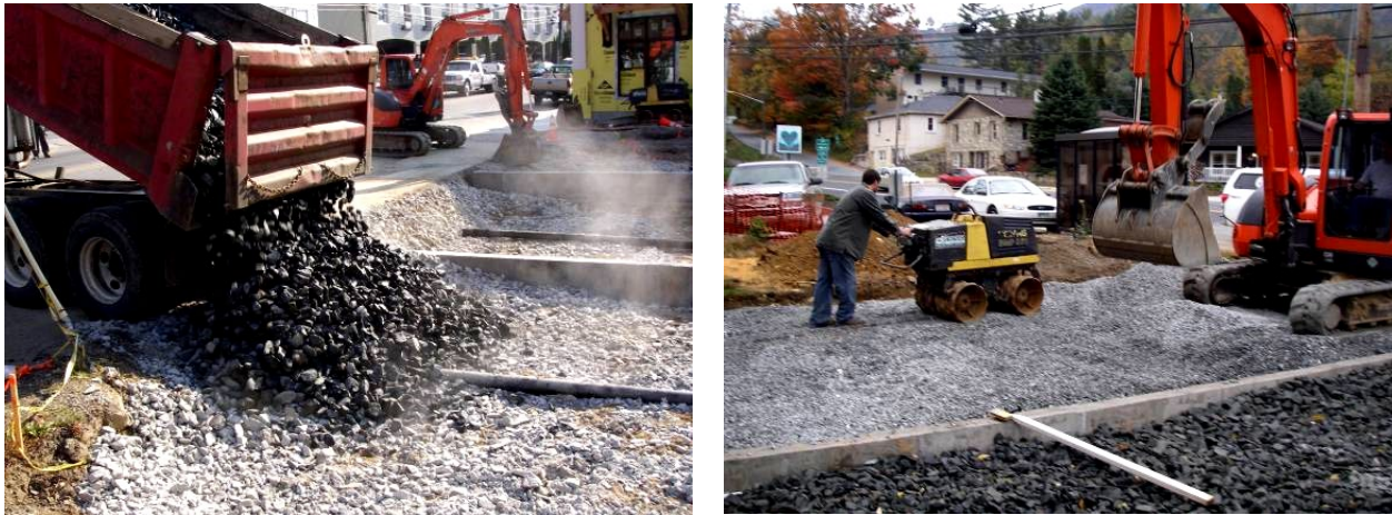
Figure 12. Aggregate Placement and Compaction (NCSU-BAE)
