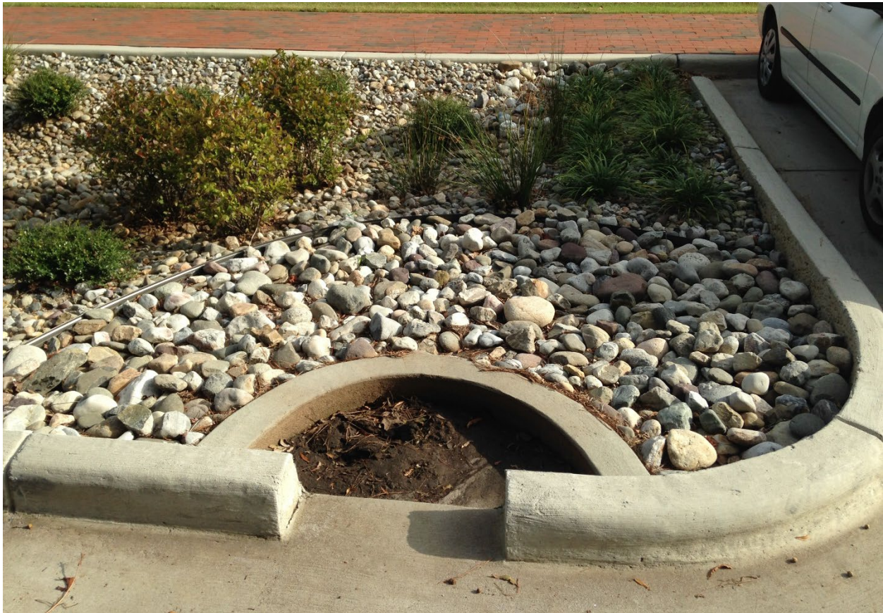
Figure 4: Example of Concrete-Lined Bioretention Forebay
