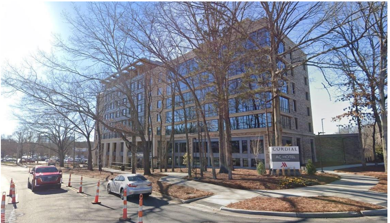
View of the AC Hotel located southeast at the corner of Rexford and Roxborough Roads.
