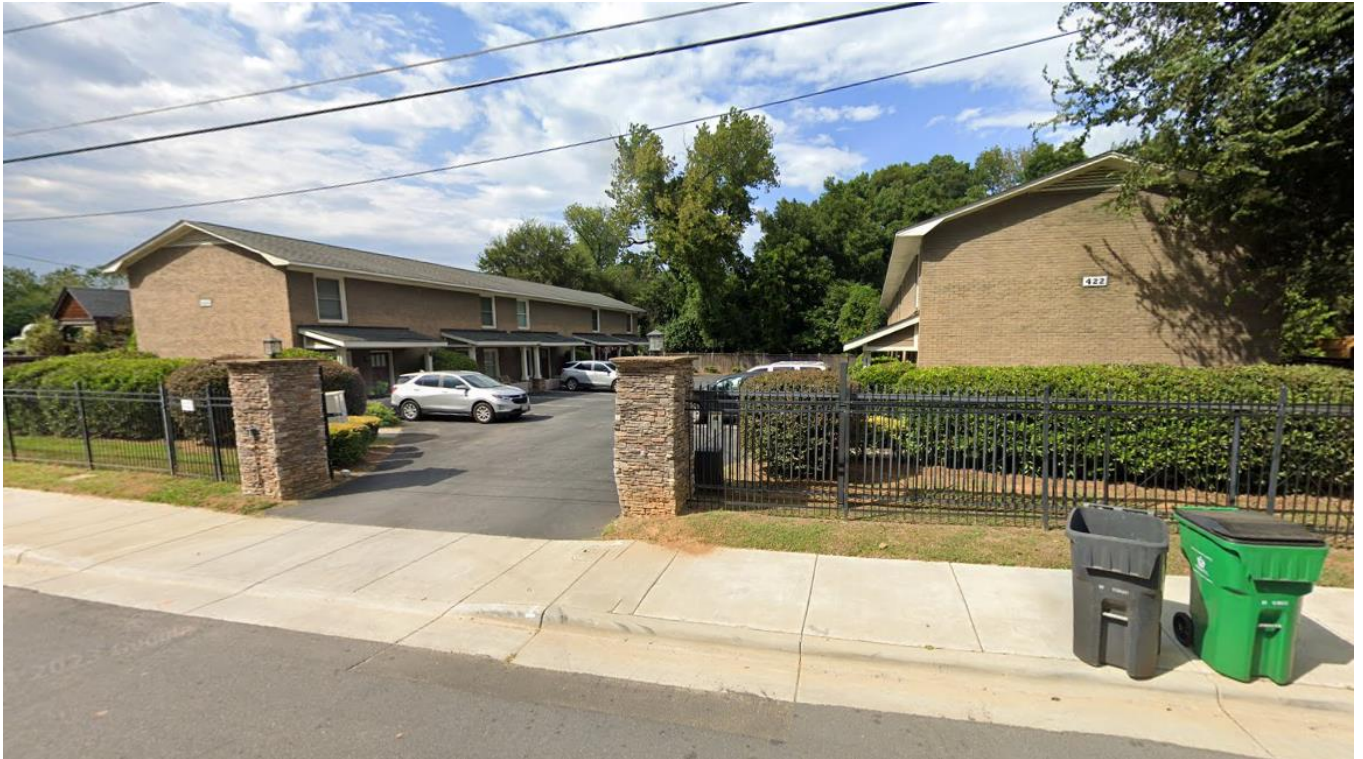
View of a multi-family development located on State Street east of the site.
