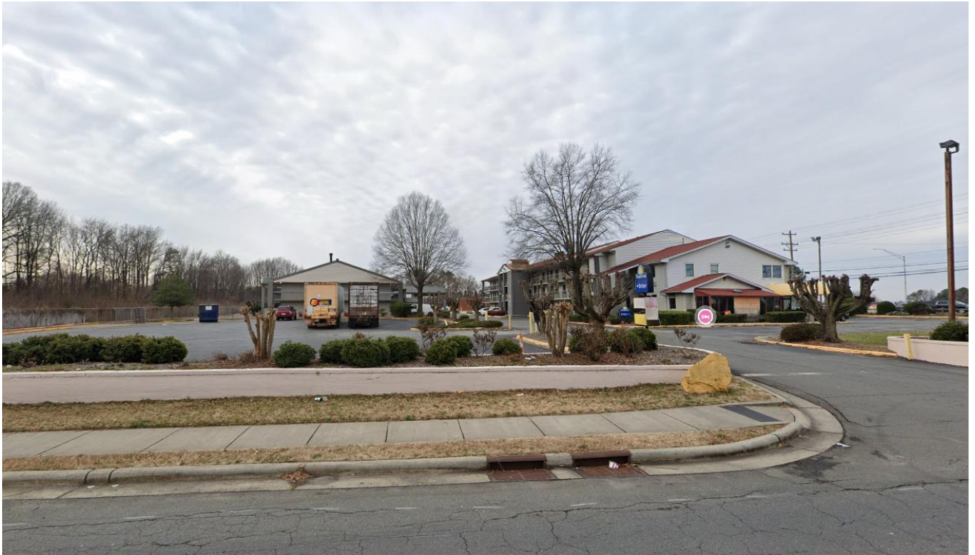
View of a motel located across Milhaven Lane, west of the site.
