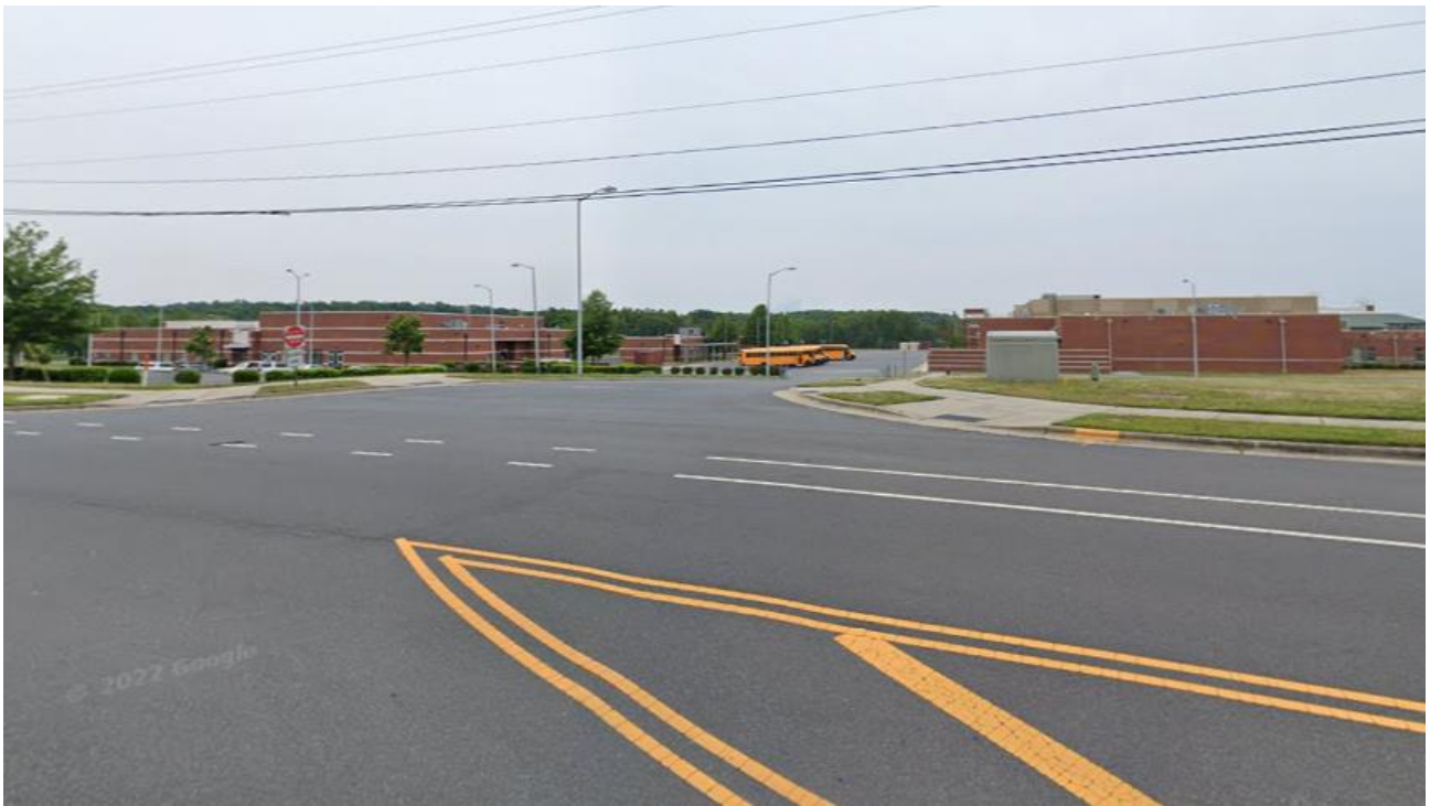
View of Whitewater Academy and Whitewater Middle schools located to the south of the site across Belmeade Drive.
