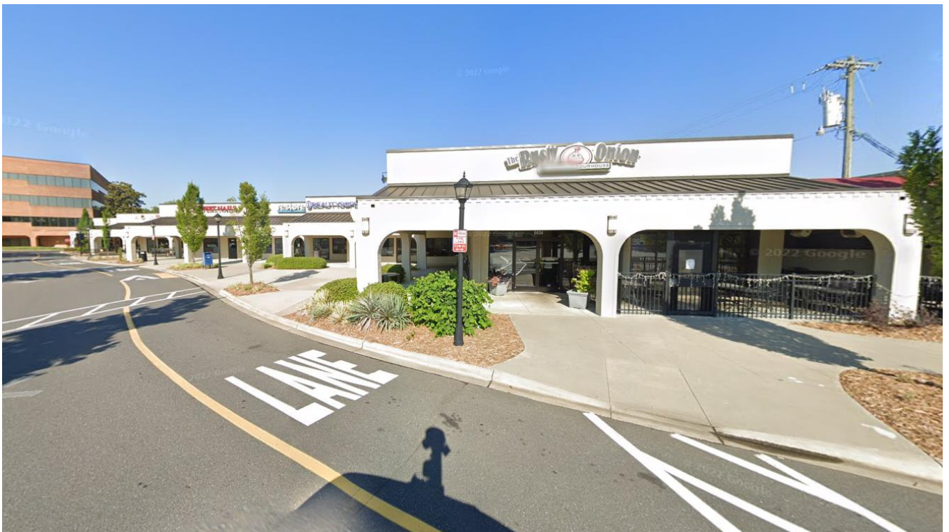
View of the Carmel Common Shopping Center containing neighborhood scale services such as retail, restaurant, and banking uses which will be directly accessible to the site via a proposed sidewalk.
