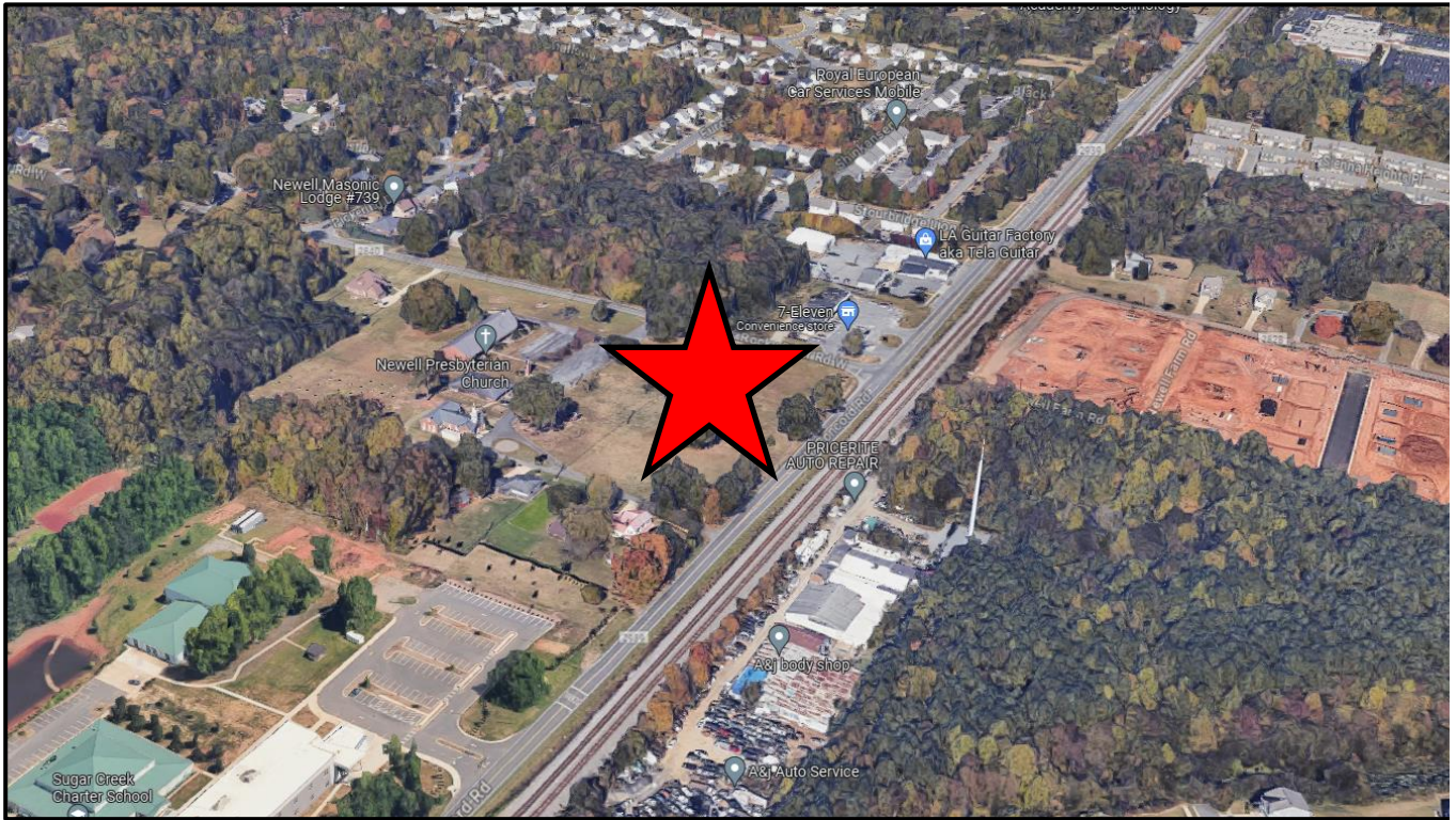
The subject property is denoted by a red star. The surrounding land use include a religious institution, a school, single family homes, multi-family apartments, commercial/retail and industrial uses.
