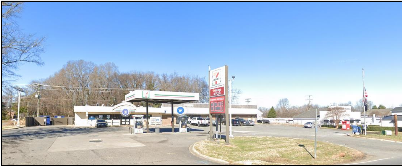
The property to the north along Old Concord Road is a 7-Eleven store.
