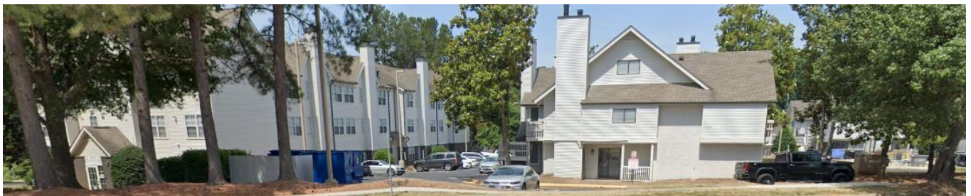
Street view of multi-family use, converted from hotel use, north of the site as seen from Westpark Drive.
