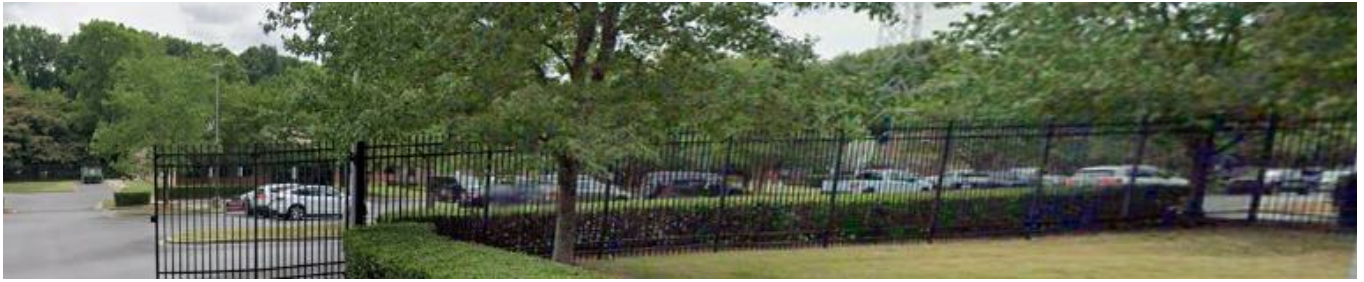
Streetview of the western portion of the site that is developed with an office building as seen from Wood Ridge Center Drive.
