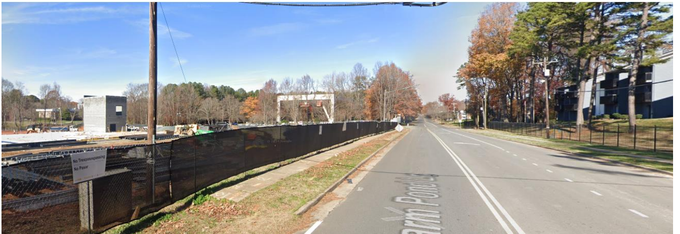
South are an educational campus under construction, office, and multi-family residential units.
