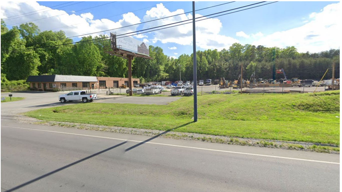
View of a construction equipment and storage yard to the south of the site along Brookshire Blvd.
