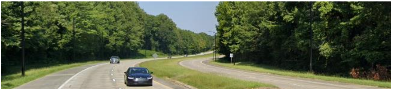
Billy Graham Parkway is immediately north of the site.
