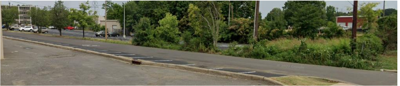
Street view of the site, developed with a parking lot and small warehouse, as seen from Wallingford Street.
