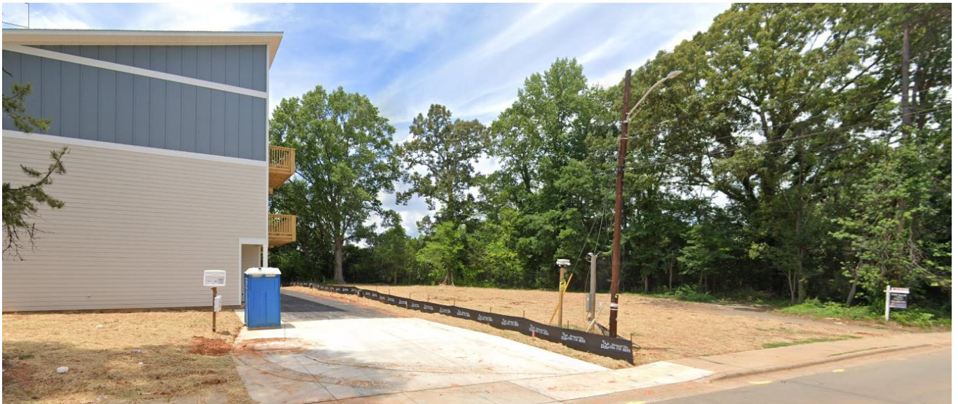
West are townhomes under construction.
