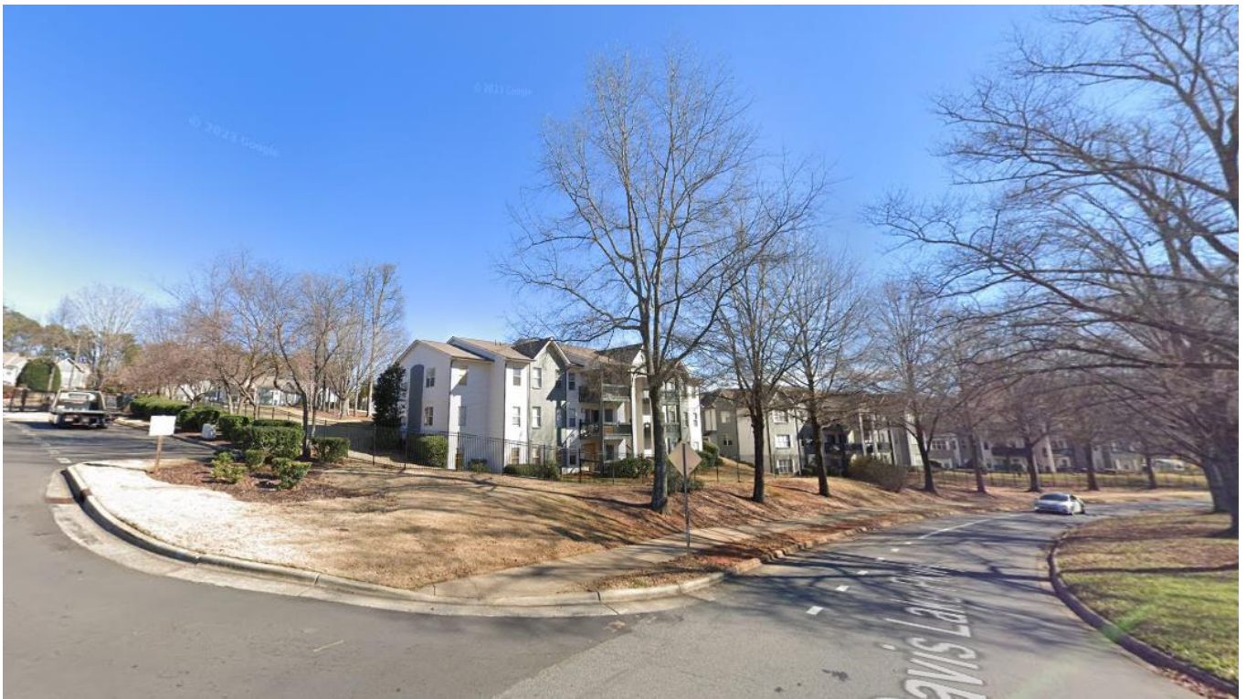
View of a multi-family development located to the east of the site across Davis Lake Pkwy.
