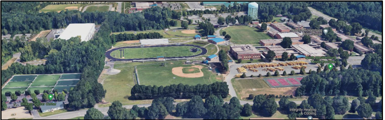
The property to the north and northwest of the site along Alexandrina Road is a Strikers Soccer Center and North Mecklenburg High in Huntersville.
