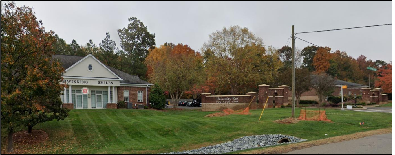
The property to the north along East WT Harris Boulevard is the University East Business Park.
