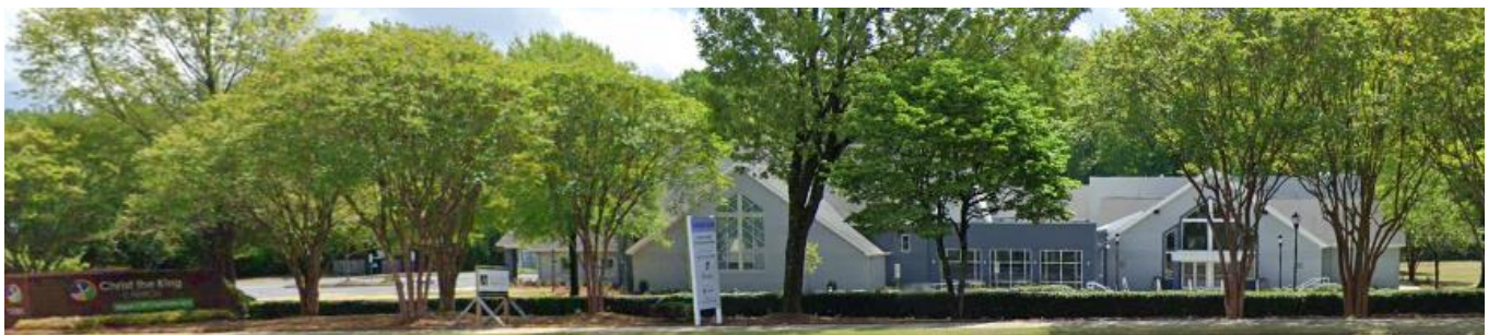
Street view of an institutional use to the north of the site along S Tryon Street.
