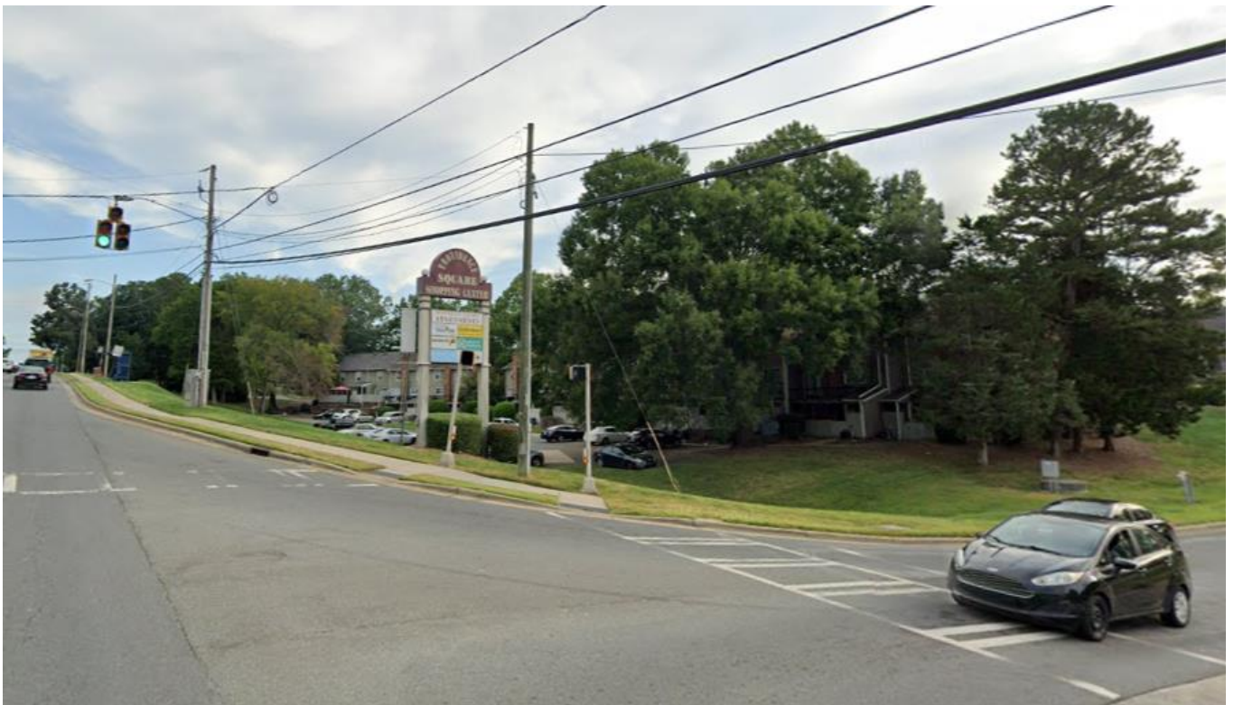
View of the Providence Square Shopping Center and Crest on Providence apartments located on the east side of Providence Road south of Sardis Lane. Looking north from the intersection of International Drive east of the site. This development is currently in the rezoning process, petition 2023-038.
