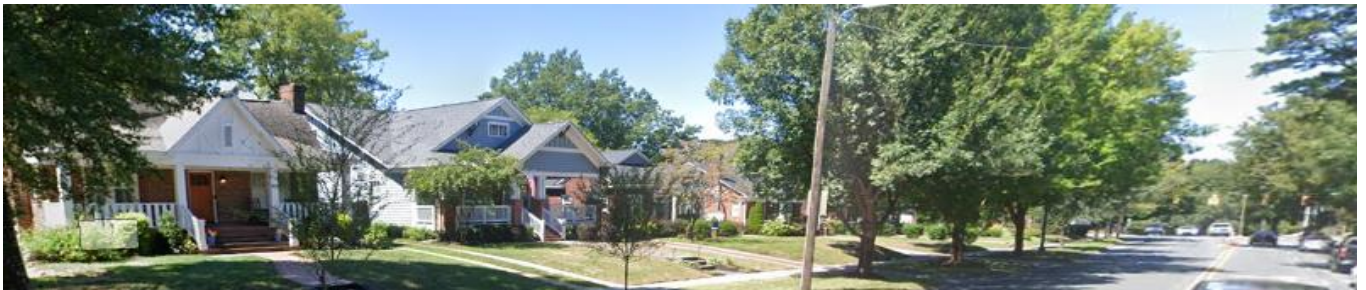
Street view of single-family residential use to the south of the site across West Boulevard.
