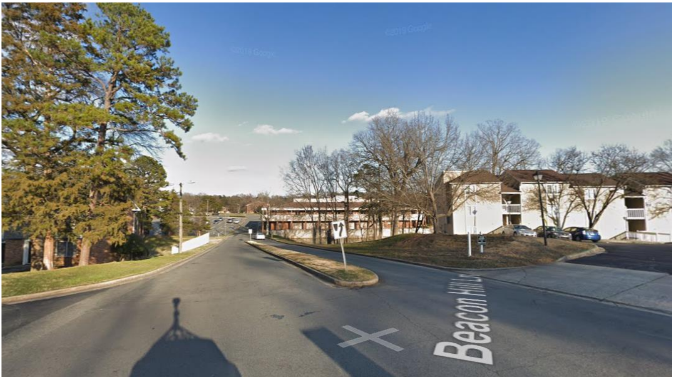
View of the commercial portion of the site from International Drive. The site contains approximate 49,000 square feet of existing commercial development.
