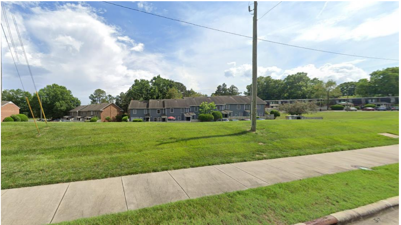
View of the site looking south from Sardis Lane. The majority of the site is developed as garden-style multi-family dwellings.
