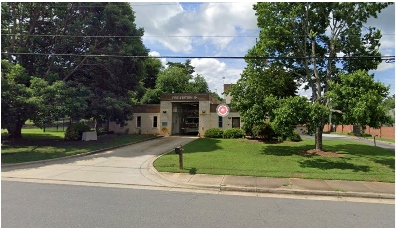
View of the Charlotte Fire Department Station number 19 on Sardis Lane, located adjacent to the site.
