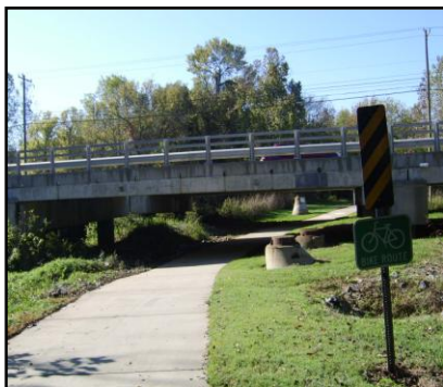
Mallard Creek Greenway crossing under North Tryon Street/US-29.
