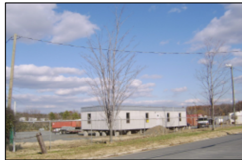
Industrial area located on Raleigh Street within the Light Rail Alternative – Sugar Creek Design Option alignment that would be subject to partial and full acquisitions, resulting in business displacements.
