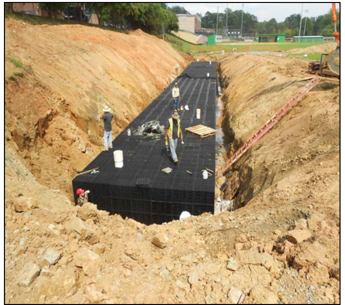
Figure 3: Installation of the 15,000 cubic foot infiltration water storage device.
