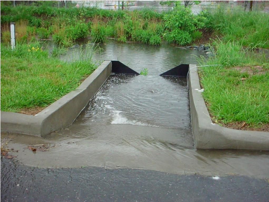
**Figure 2.** 120° weir at the HMBC inlet.
