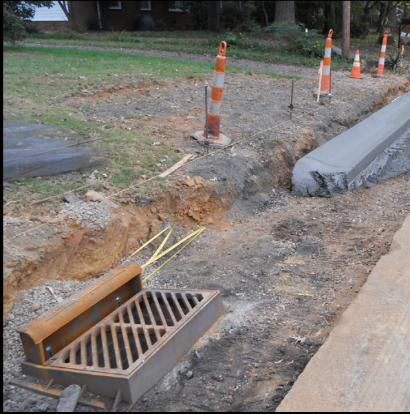
Concrete curb and gutter is being installed along Woodbridge Road.
