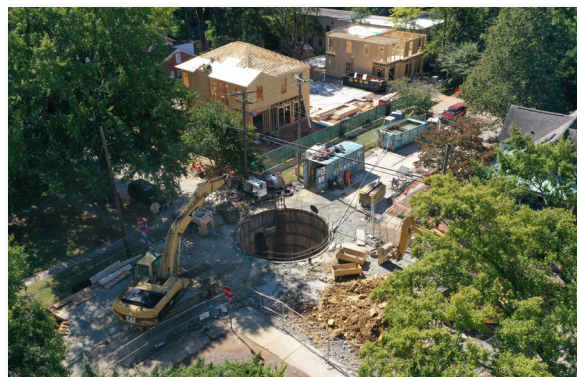
Tunneling operation for installation of 84-inch stormwater pipe on Lexington Avenue.
