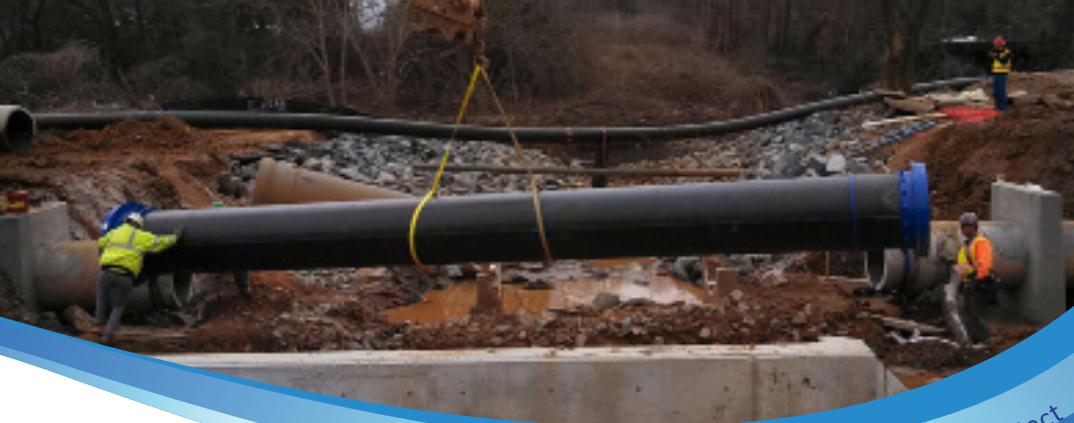
Greenhaven/Pierson Storm Drainage Improvement Project
