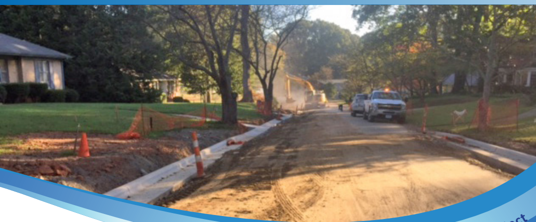
Photo: Contractor works on Chillingworth Drive.
