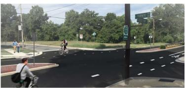
Wheelchair ramps are complete on the north end of Rozzelles Ferry Road, with the contractor working to remove and reinstall the new wheelchair ramps on the south side. Construction will also include pedestrian refuge medians, street resurfacing, drainage improvements, landscaping and street trees.
