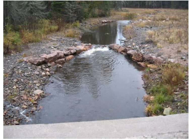
PHOTO: CROSS VANE PLAN VIEW
