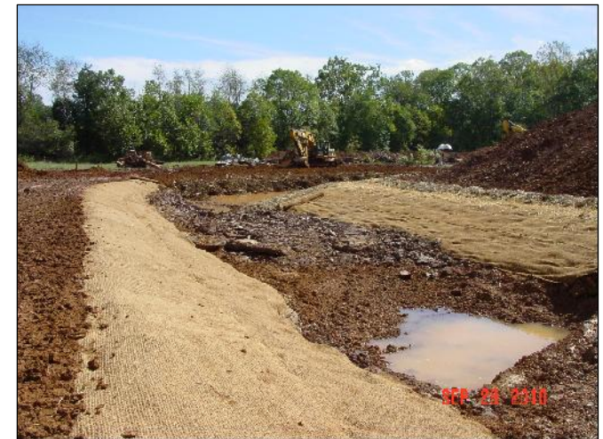
PHOTO: VARIABLE RIFFLE UNDER CONSTRUCTION
