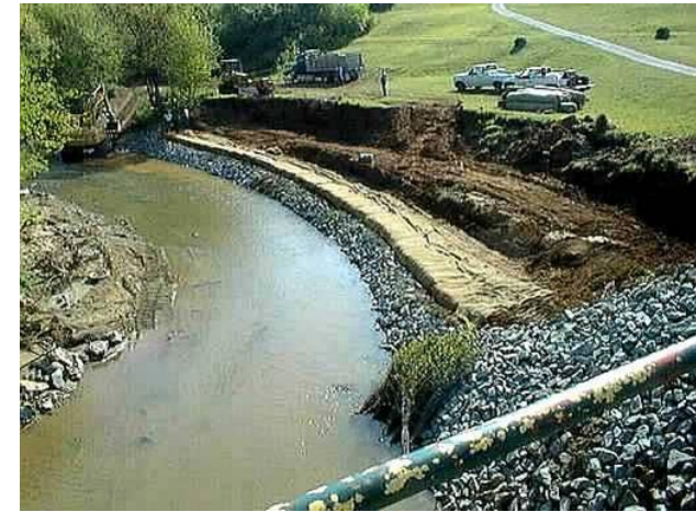
PHOTO: VEGETATED GEOGRID UNDER CONSTRUCTION
