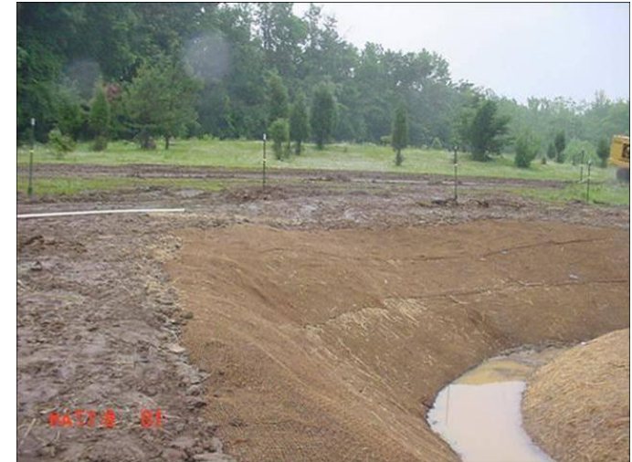
PHOTO: EROSION CONTROL MATTING ON STREAM BANK
