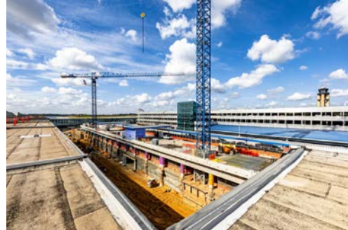
Charlotte-Douglas International Airport
