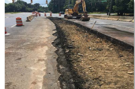
Intersection & Roadway Improvement
